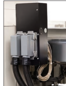
Quick change heater disconnects
